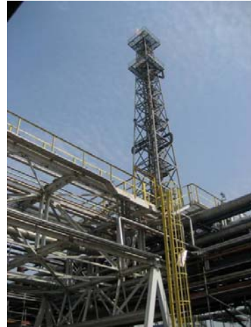
Typical structure inspected
